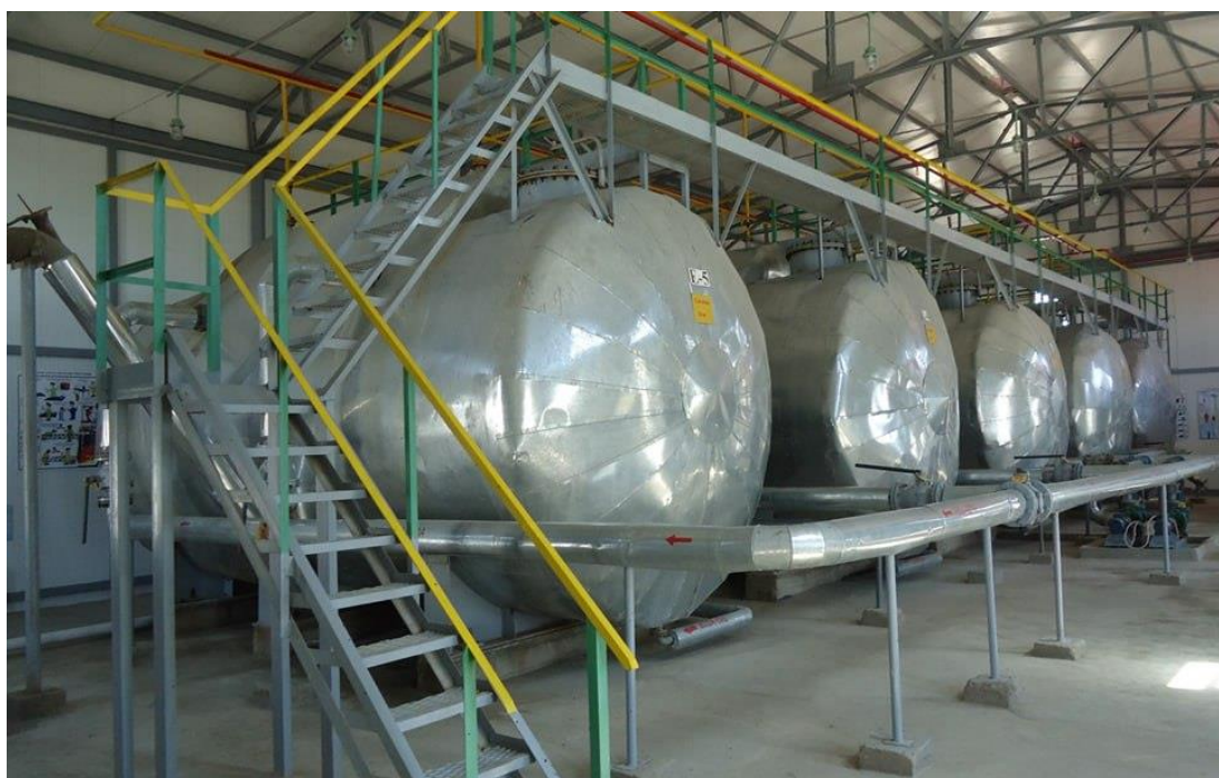
2-rasm. Biogaz ishlab chiqarish bioreaktori
