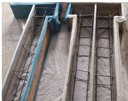
Picture 2. Preparation of reinforcement frames and placement in molds.
